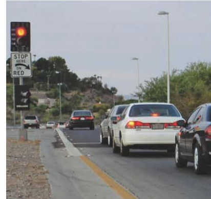
Typical ramp meter
